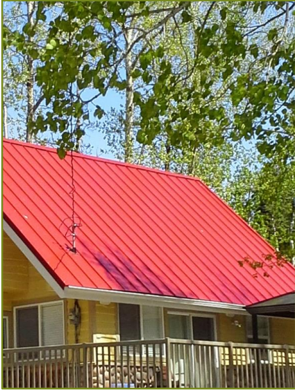
Figure 19. Tin roofing
