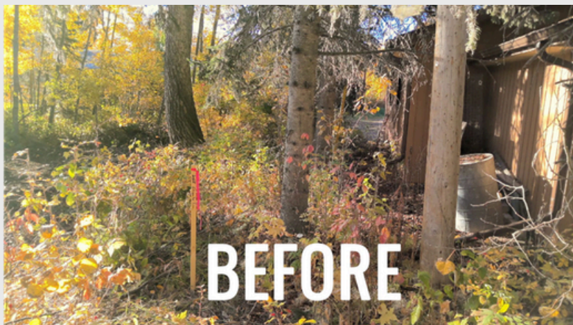
Figure 7- Before Brushing and Tree Removal
