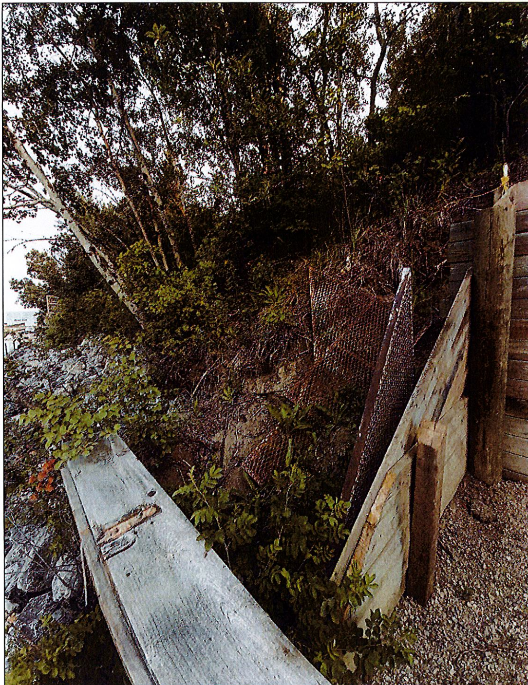
Photograph No. 3: Photograph taken from near the toe of the slope, within the historic deck footprint, facing northwest, showing evidence of recent slope movement. Photograph taken on the 16 th July, 2021.
