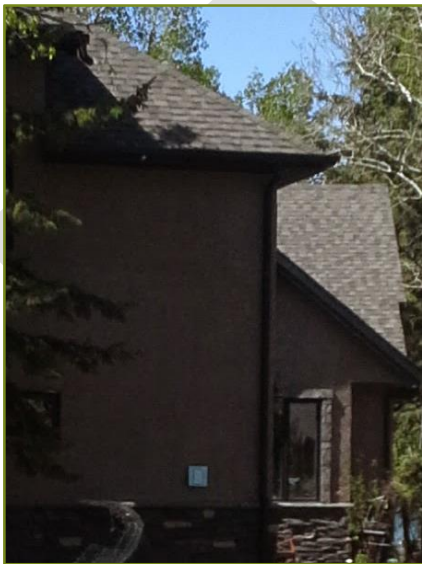
Figure 21. Stucco siding
